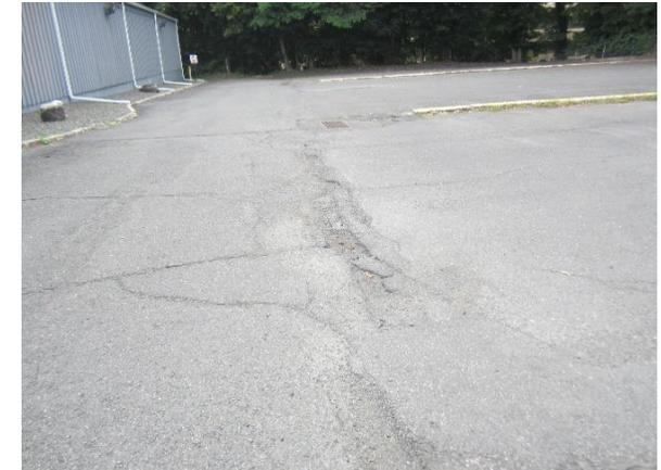
This site contains a building that has disconnected downspouts on both sides of it. The driveway is highly eroded and could benefit from pervious pavement. Porous asphalt can be used to replace the existing driveway and parking spaces north of the building to capture and infiltrate stormwater generated by the building and parking lot. A preliminary soil assessment suggests that the soils have suitable drainage characteristics for green infrastructure
